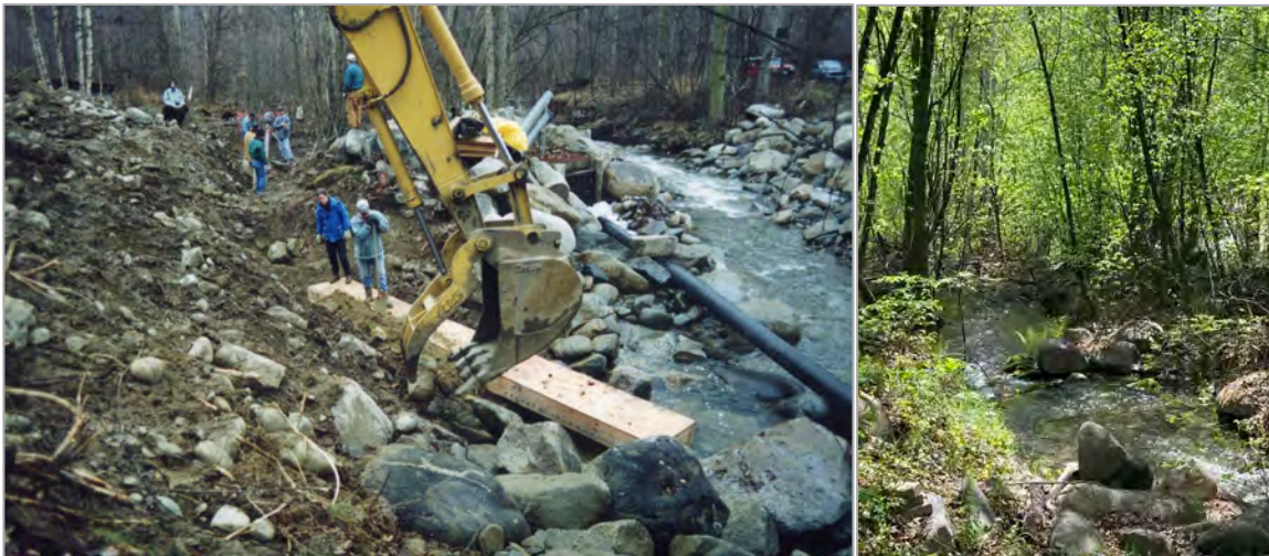
Figure 12. Murphy Creek spawning channel undergoes expansion in 2000 (left); the naturalized spawning channels in 2021 (right; photo by Al Mallette).
