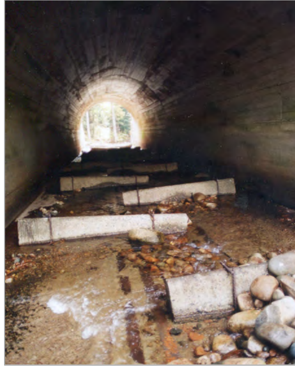
Figure 13. The Blueberry Creek culvert fish passage bars were installed in 1998.
